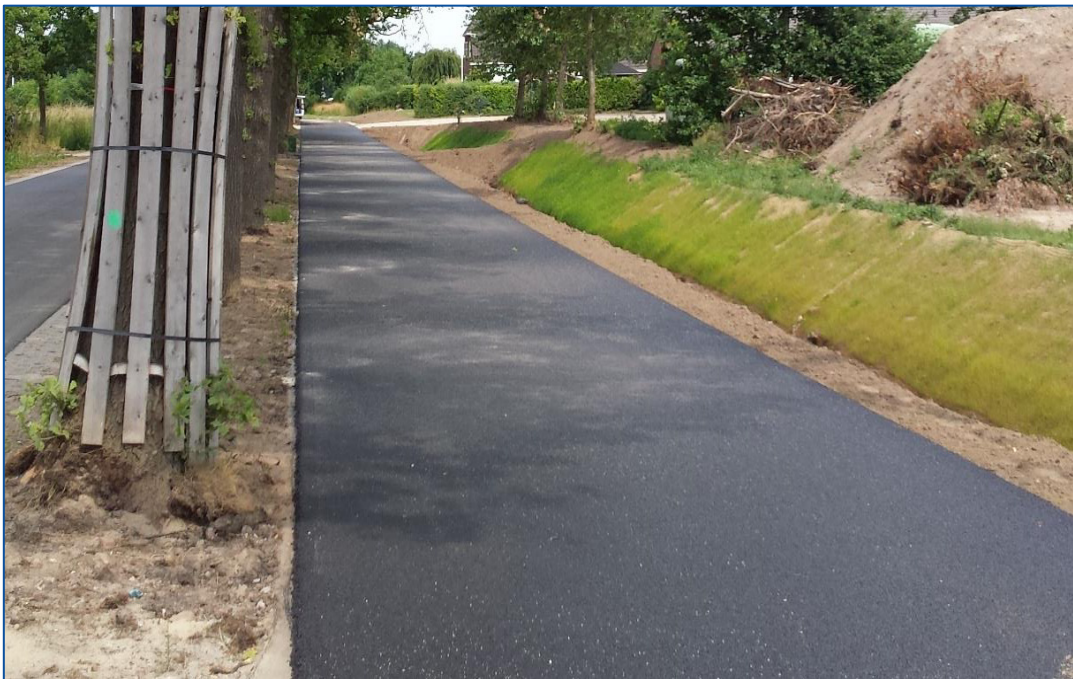
Figure 3. 2 Cycling path paved with lignin-based asphalt at Wageningen campus in 2017
