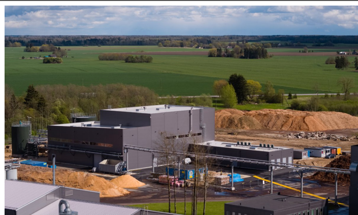
Flagship plant in Estonia, Imavere
